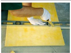
Absorptive material was applied to the walls from floor to ceiling beside and behind the speakers and along one side wall.
