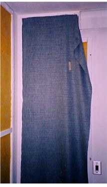
Here's a word to the frugal. Commercial sounddamping products are surprisingly expensive and none are more effective than the compressed fiberglass material that I used which is cheap and readily available from builders' supply stores everywhere. Most commercial products actually use the same or equivalent compressed fiberglass
